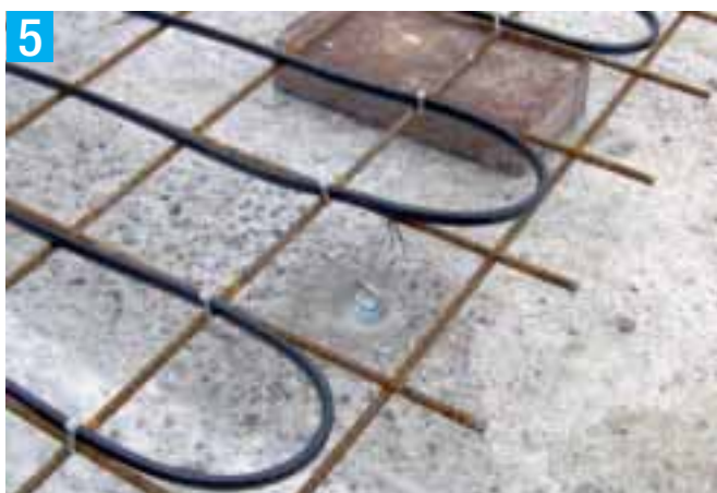
5) Particolare del fissaggio tramite fascette Detail of the panel mounting by clamps
